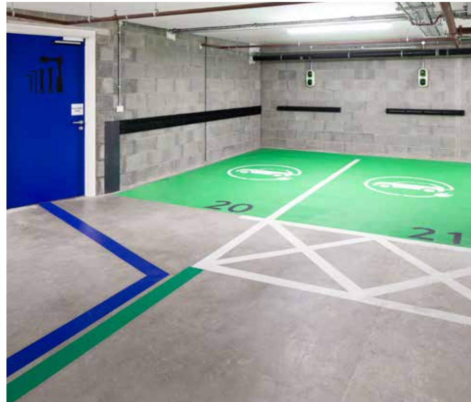
Electric car charging points
